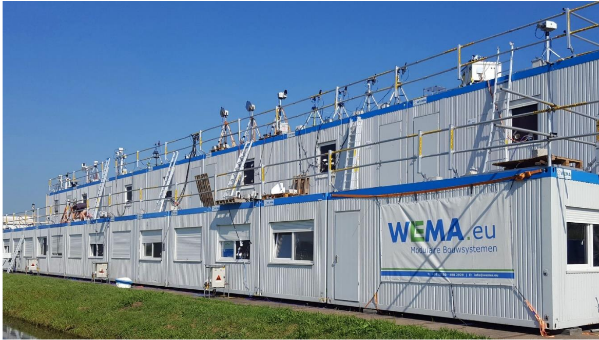
Figure 2: The CINDI-2 container layout at the CESAR Remote-Sensing Site (RSS). The picture shows the organisation of the MAX-DOAS instruments on two superposed rows of containers.
